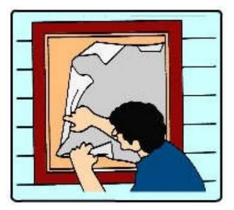
The residual film should be removed immediately after the glazing is completed.
